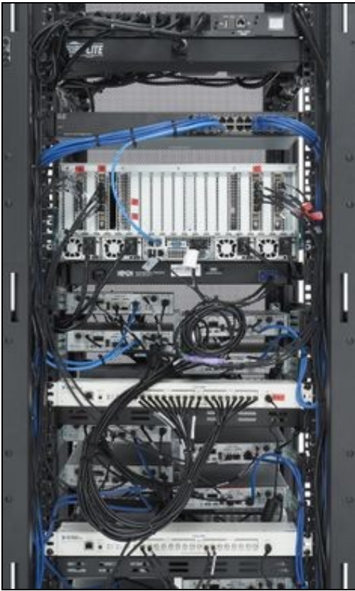
Figure 8. Rack Layout for 32x32 System
